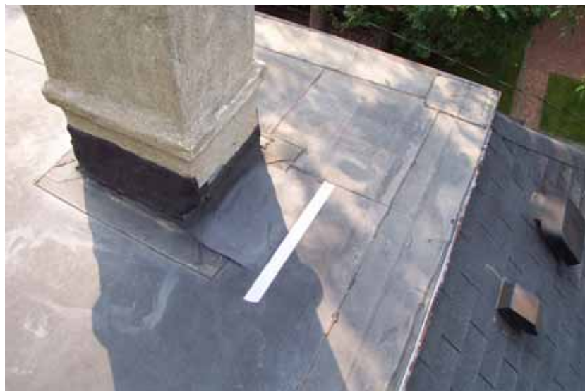
TEAR (#2) IN RUBBER MEMBRANE
