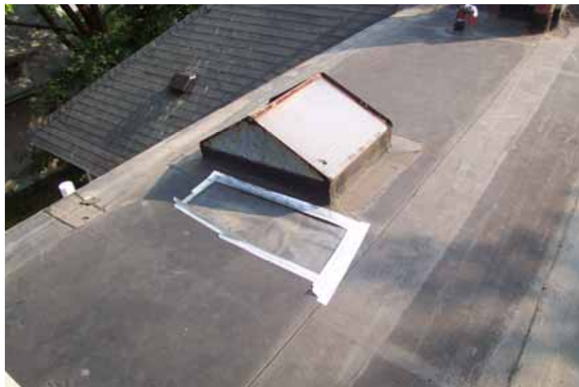
TEAR (#2) IN RUBBER MEMBRANE
